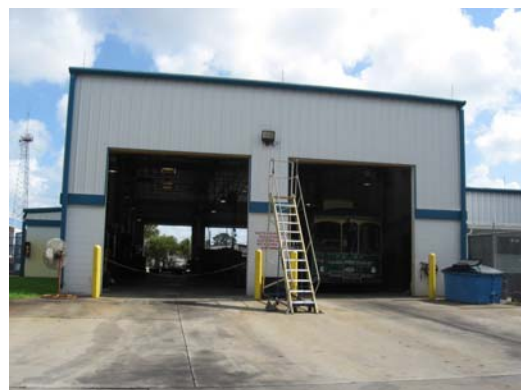
Maintenance bay at the north terminal.
